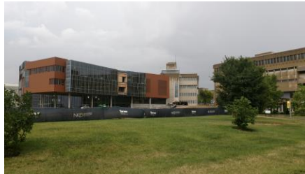
Founders Hall with the new Health Innovation Center, Kenton Drive side
